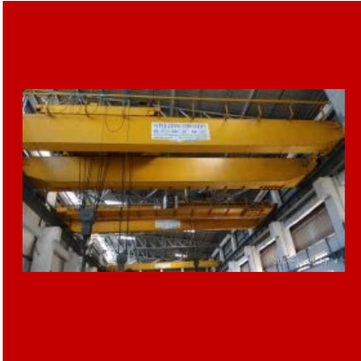
Material Lifting Cranes
